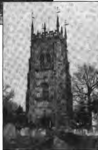
GREAT TOWER OF EVESHAM ABBEY (Actual Condition)
